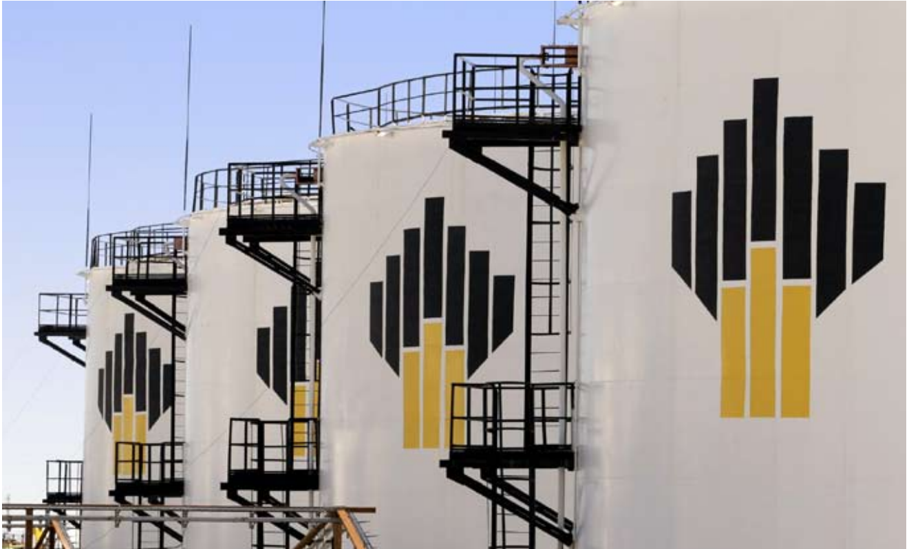
Purneftegaz fuel and lubricants base – tank farm
